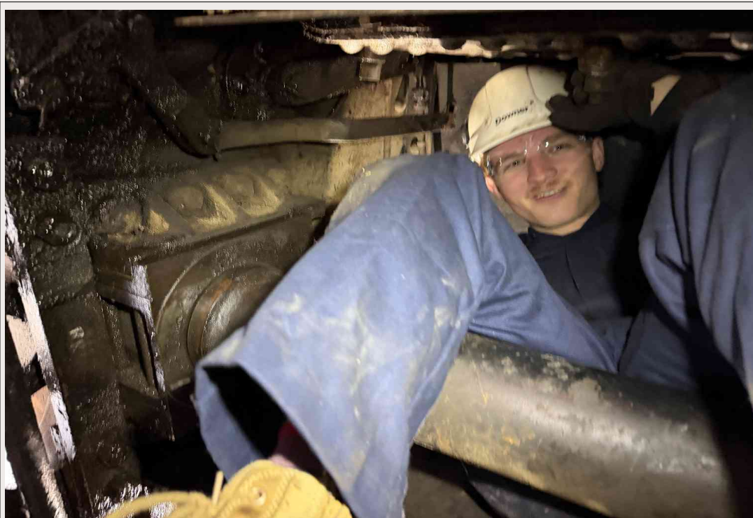
Above: Evan W installs Peckett springs in a very confined space (GuyC)
