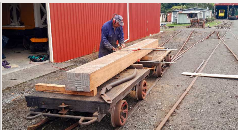
Above & Right: Heisler headstocks preparation: firstly careful cutting of the large yellow heart baulk, then drilling holes for mounts (with steel bands fitted) (JS)
