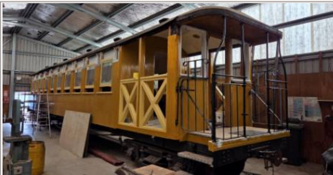
Above: A1477 showing works above windows & end verandah (Richard E)
