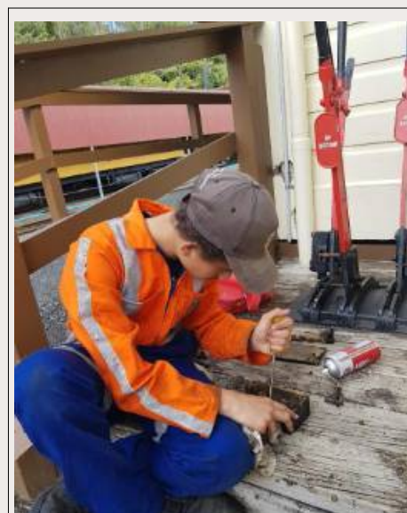
Above: repairs by JD (Florina B)
